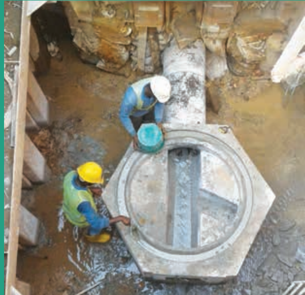
◆ Sewer rehabilitation project works at Sri Lanka
