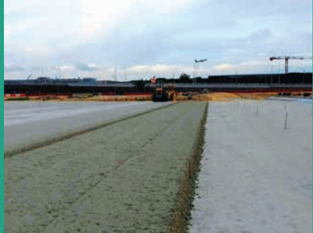
◆ Supply and lay of aggregate road base for airport taxiway
