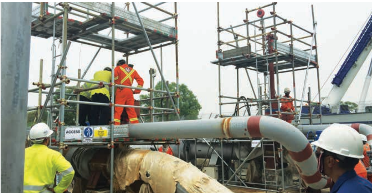
◆ Natural Gas pipeline installation works.
