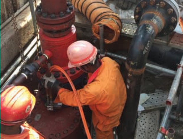
◆ Natural Gas pipeline installation works
